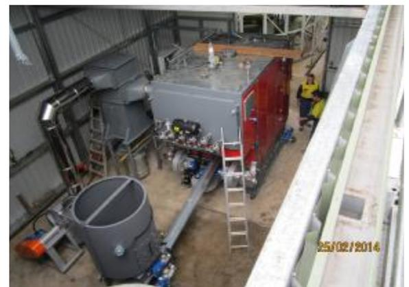
Right—The shell fired boiler used to supply all the heat energy for drying.
